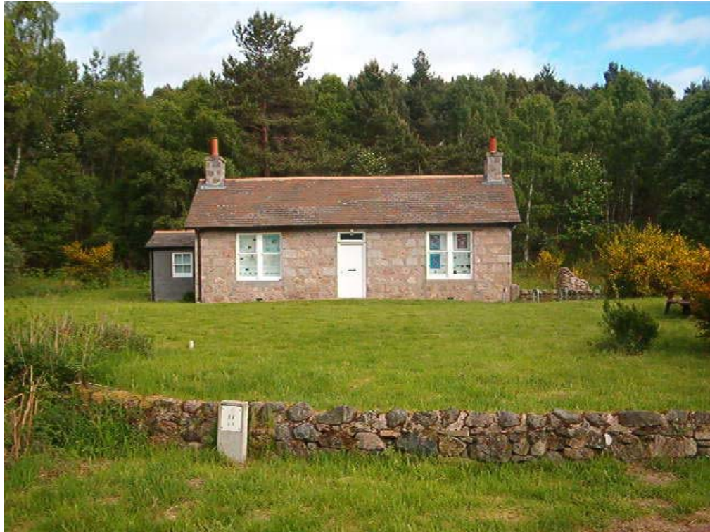
Fig. 3. Existing Visitor Centre Building from the B9119
